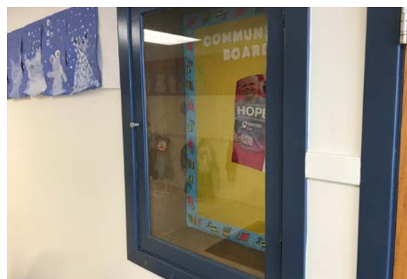
Fire Extinguisher Cabinet
