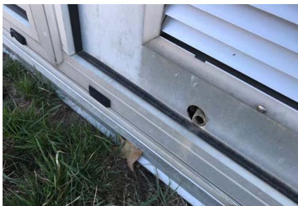
Unit Vent Drain (typical)
