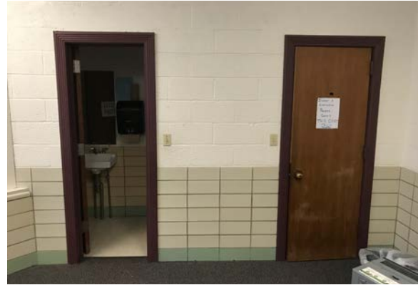
Bathroom (Area A)
