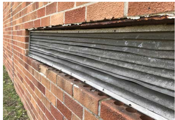
Louver (corrosion)
