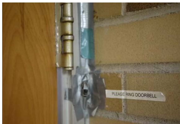
Exterior Classroom Doorbell
