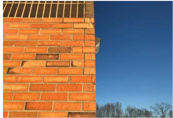
Brick (cracking)
