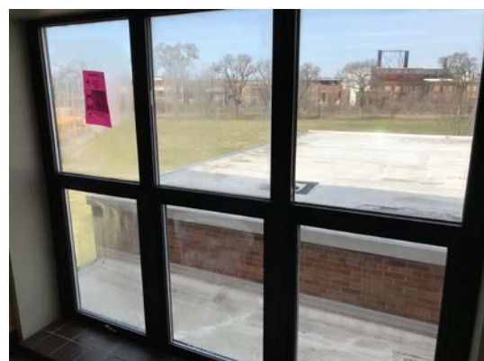
2nd Floor Windows
